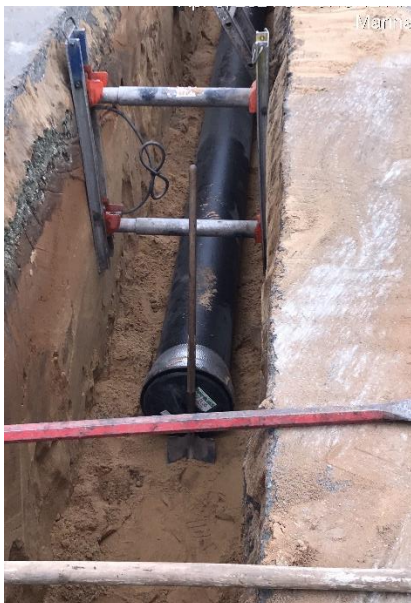
Ductile iron pipe in trench
