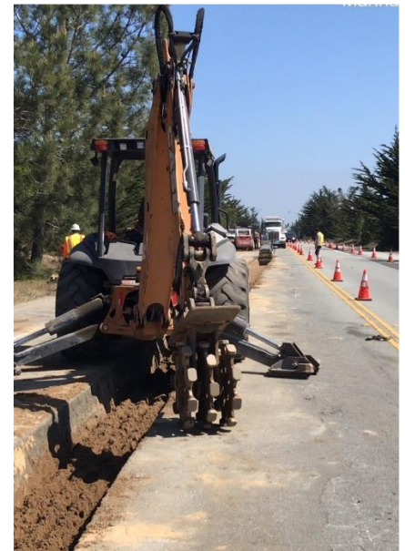
"Sheep's foot" compaction attachment
